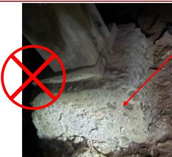
EFFLORESCENCE DEVELOPS AS AN INDICATOR OF INTERNAL LOSS OF BOND. DETERIORATION & SPALLING ENSUES
